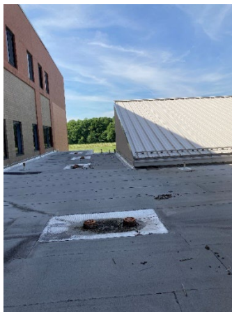
Monroe Twp. High School – Building Envelope
