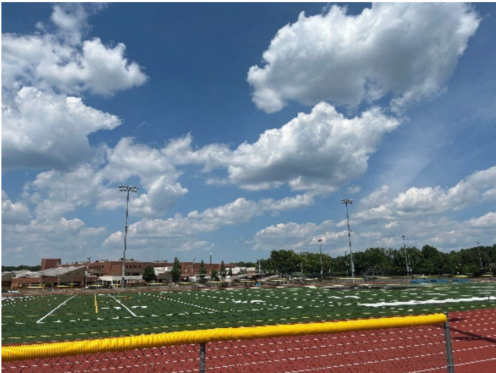
Sports Field – Stadium Lighting
