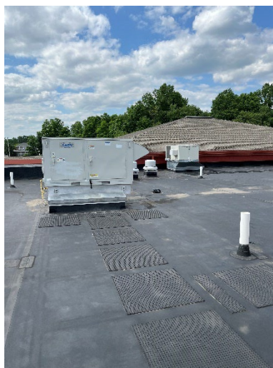
Brookside School – Existing Roof
