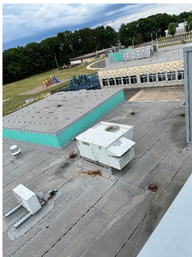
Mill Lake School Complex– Existing Roof
