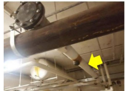
Uninsulated hot water piping
