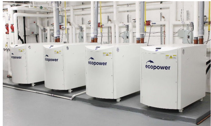
4.4kW Micro-combined CHP
