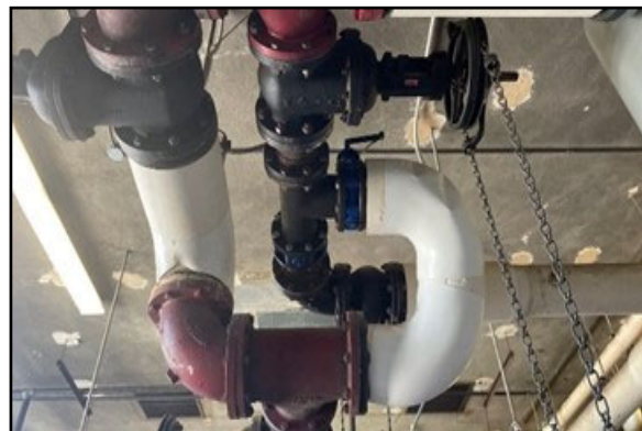
Uninsulated hot water piping
