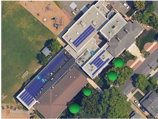
Potential Roof Mount Solar - Elizabeth Haddon ES
