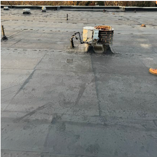
Haddonfield Memorial High School – Existing Roof
