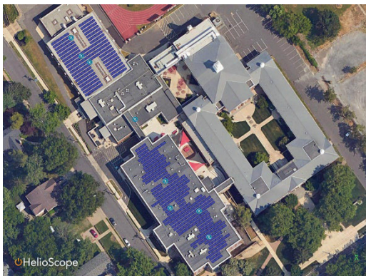
Potential Roof Mount Solar - Haddonfield HS
