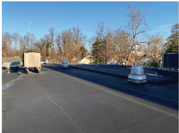
J. Fithian Tatem Elementary School – Existing Roof
