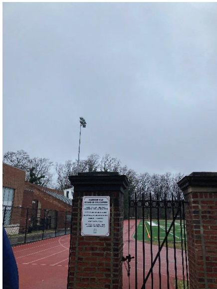
Haddonfield Memorial High School – Stadium Lighting
