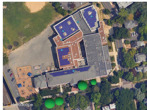
Potential Roof Mount Solar – Haddonfield MS
