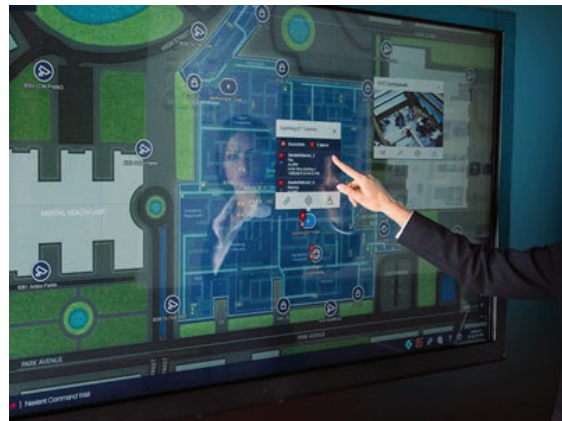
HVAC Equipment Control
