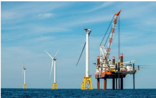
Figure 16-2: Turbine installation at Block Island wind farm (top left), representative turbine installation vessel (Seajacks Ltd.) (top right), representative transport barge vessel 179 (bottom left), representative CTV 180 (bottom right)
