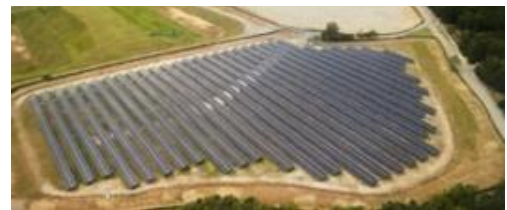
Figure 1-9: 30 MW solar project at former Ciba Giegy superfund site
