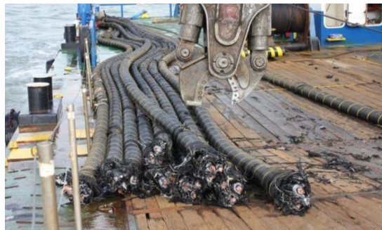
Figure 16-4: Example tracked jet plow 182 (top left), hydraulic cutting of power cables (top right), representative construction support vessel 183 (bottom left), representative crane barge for cables 184 (bottom right)
