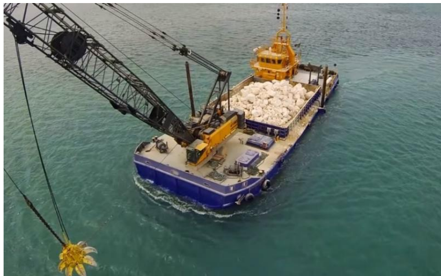
Figure 16-6: Representative crane barge for scour protection removal 186
