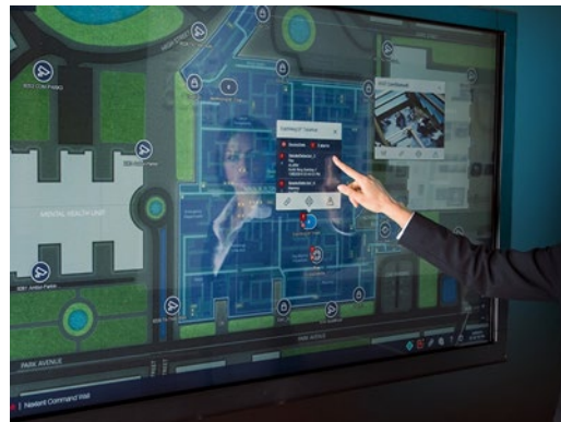
HVAC Equipment Control
