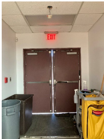
Rosa Parks Community School - Building Envelope
