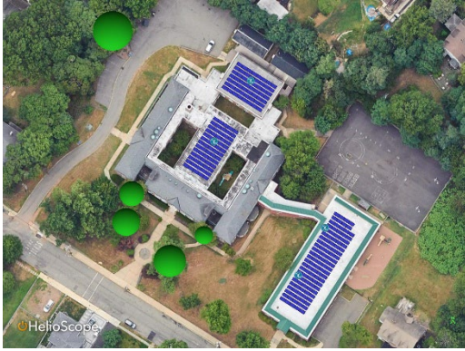
Heywood Avenue School – Solar PPA
