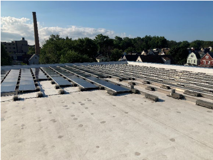
Lincoln Avenue School – Existing Roof
