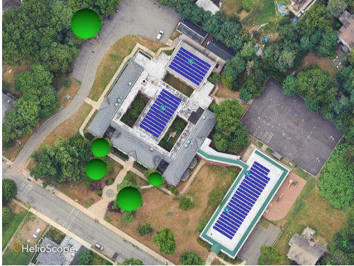
Heywood Avenue School – Solar PPA
