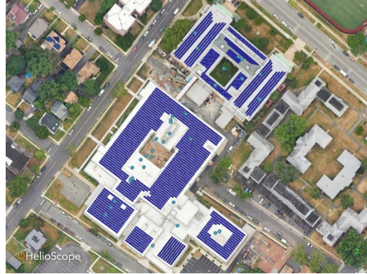
Orange High School and Prep Academy – Solar PPA
