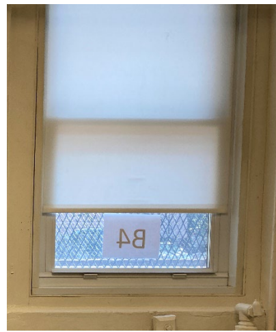
Country Club Administration Building - Existing Windows
