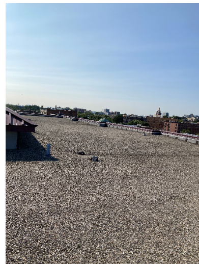
Rosa Parks Community School – Existing Roof
