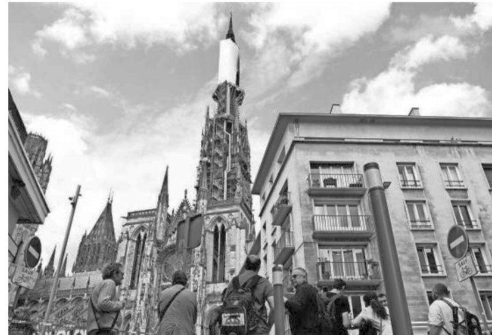
People look at the Notre-Dame de Rouen Cathedral after its spire caught fire during renovation works, in Rouen, France, Thursday. KEVIN COOMBS/REUTERS
