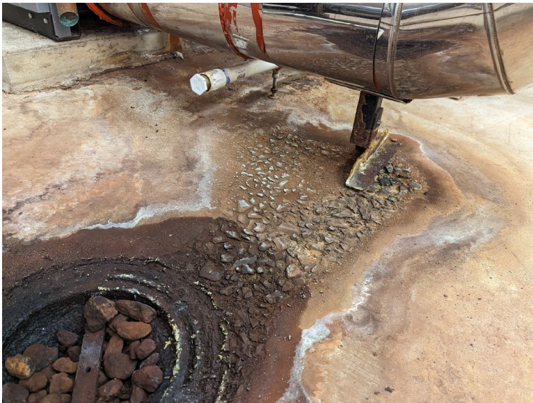
Damage from boiler stack condensate seen at each condensing boiler and floor drain.
