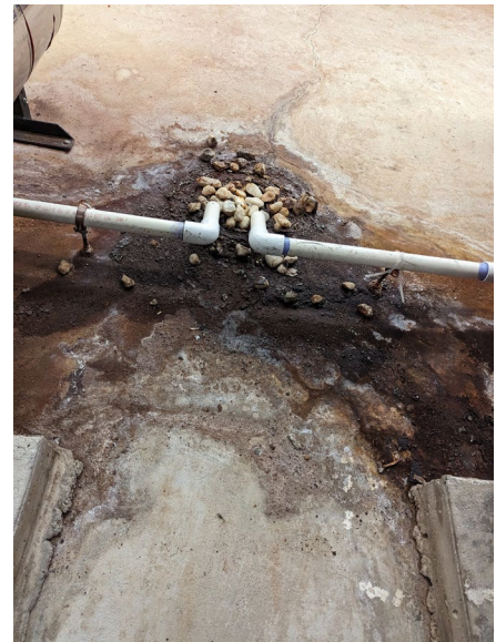
Damage from boiler stack condensate seen at each condensing boiler and floor drain.
