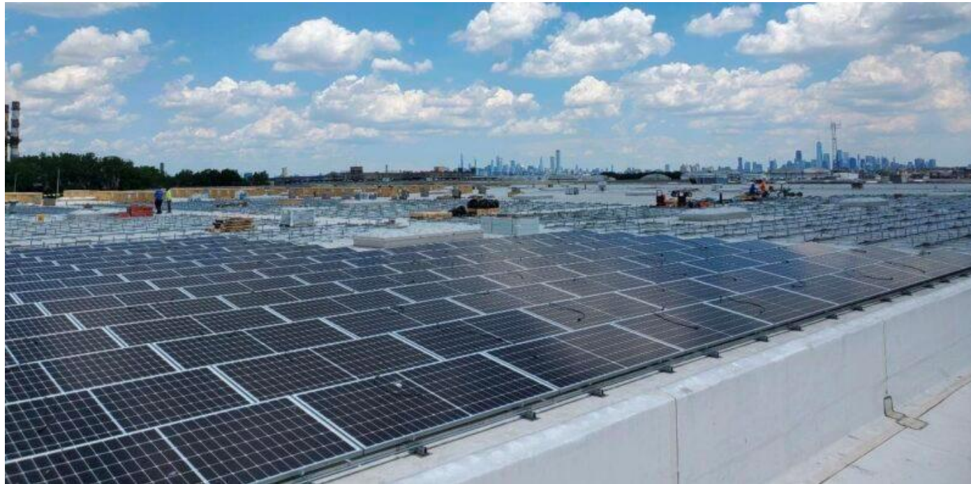
Caven Point, Jersey City – Photo Courtesy Hartz Mountain/PowerMarket
