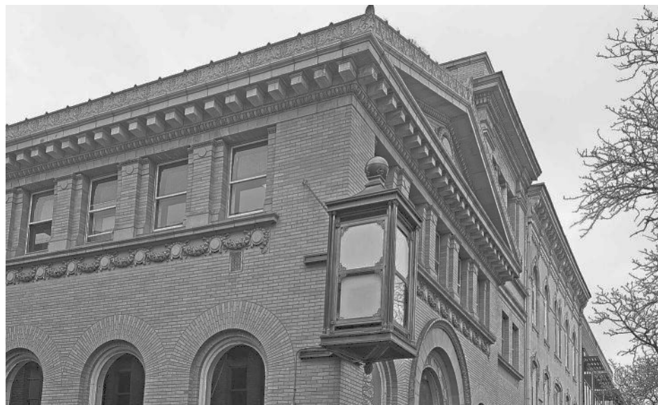
The century-old bank building on West Main Street in Somerville will be transformed into a vegan restaurant with a jazz theme. MIKE
