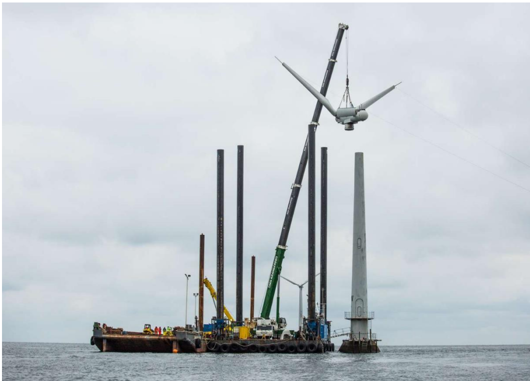
Figure 5-2: Decommissioning of Vindeby Offshore Wind Farm, Denmark (source: Ørsted).
