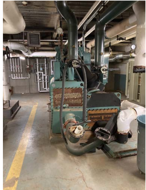
Figure 4. Non-operational Chiller
