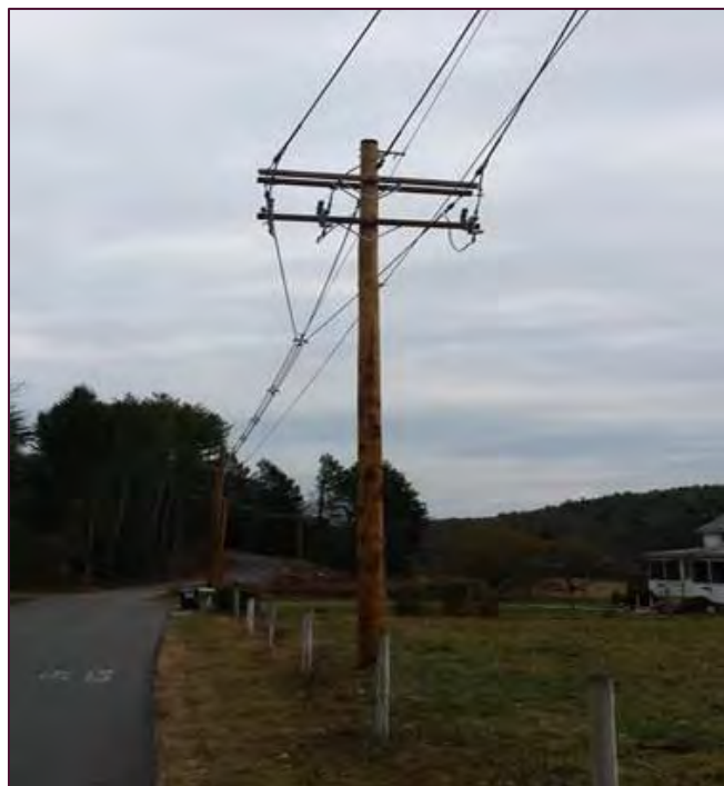
Figure 3 – Lashed Cable Photo Example
