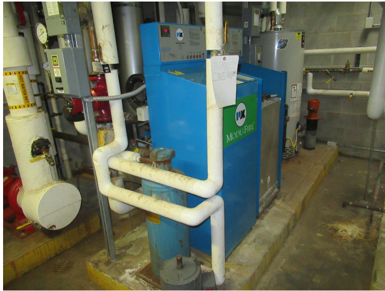
Existing non-condensing boilers at JFK Library.
