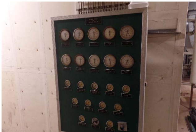
Existing pneumatics at Boardwalk & West Hall
