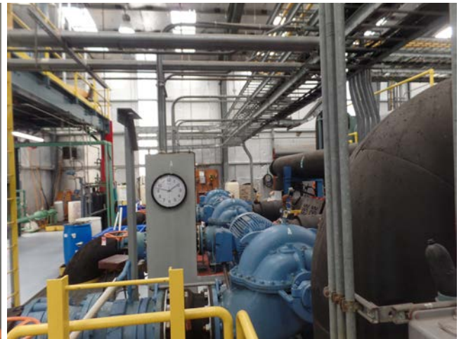
Existing thermal plant pumps
