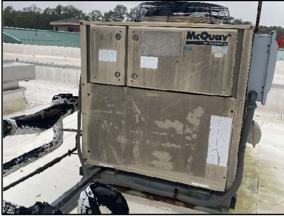
Existing split system condensers at Conover Road Elementary School and Administration Building
