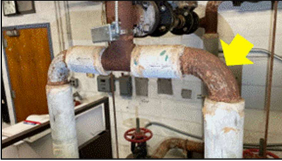
Uninsulated pipe and valves at Conover Road Elementary School and Cedar Drive Middle School
