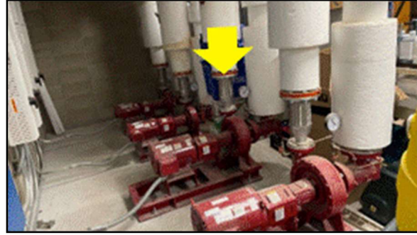
Uninsulated pipe and valves at Conover Road Elementary School and Cedar Drive Middle School
