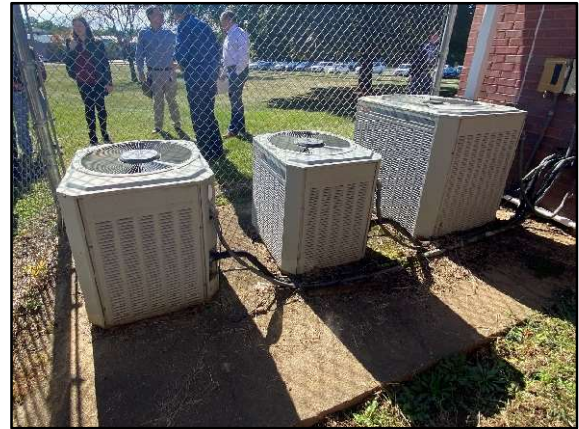
Existing split system condensers at Conover Road Elementary School and Administration Building
