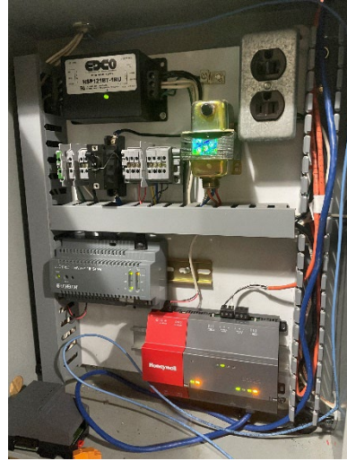
Clearview Middle School - Existing Control
