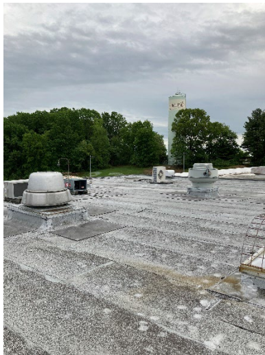
Clearview Regional High School – Existing Roof
