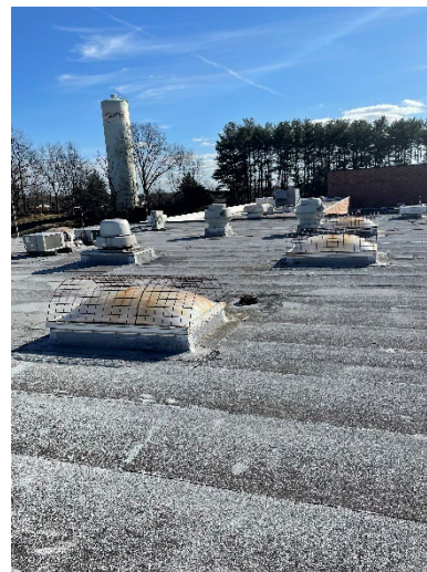
Clearview Regional HS - Building Envelope
