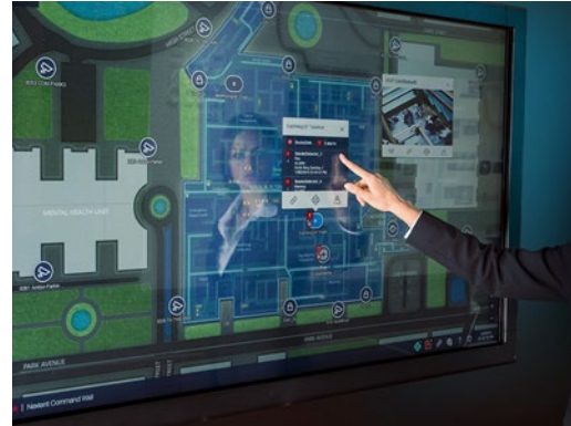
HVAC Equipment Control
