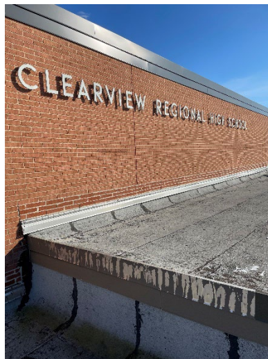
Clearview MS - Building Envelope
