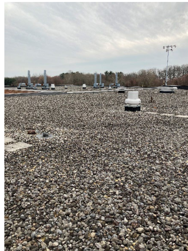
Clearview Middle School – Existing Roof
