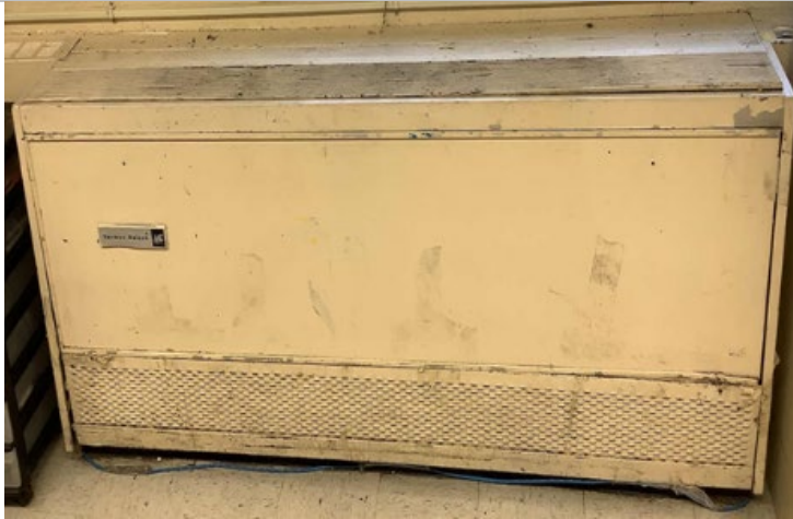
Typical Jr/Sr HS UVs, installed in 1964 or 1965.
