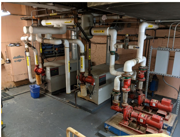
Existing non-condensing boilers at Loudenslager (left) and Billingsport (right).
