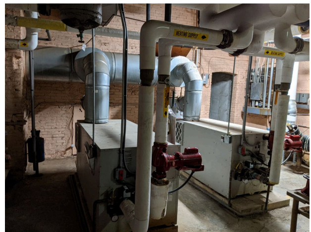
Existing non-condensing boilers at Loudenslager (left) and Billingsport (right).
