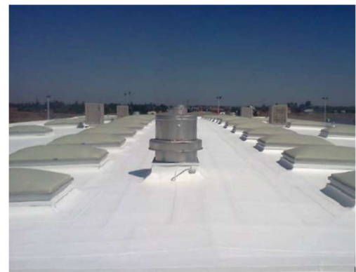
Single Ply Membrane Roof Restoration
