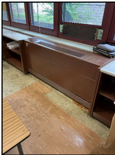
Existing Unit Ventilators at Dumont HS and Grant
