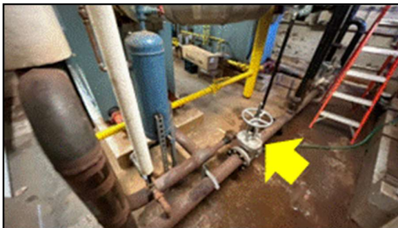
Uninsulated steam distribution and heating hot water distribution piping at Grant School and Administration Building
