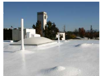
Spray polyurethane foam Roof Restoration
