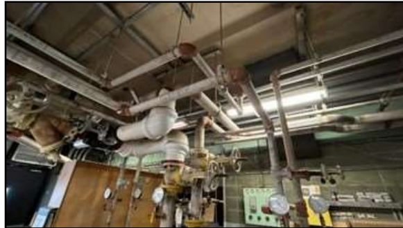
Uninsulated condensate tank and heating hot water distribution piping at Honiss and Selzer Schools.
