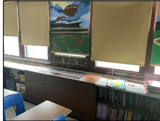
Existing unit ventilators at Selzer and Honiss
