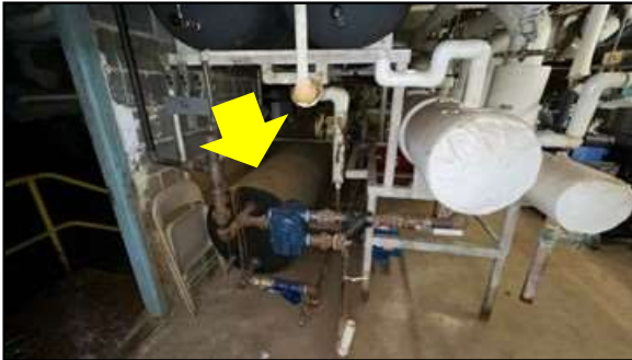
Uninsulated condensate tank and heating hot water distribution piping at Honiss and Selzer Schools.
