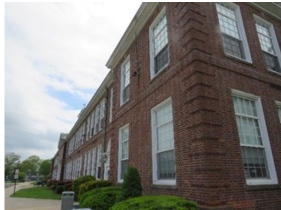
Manasquan HS - Building Envelope
