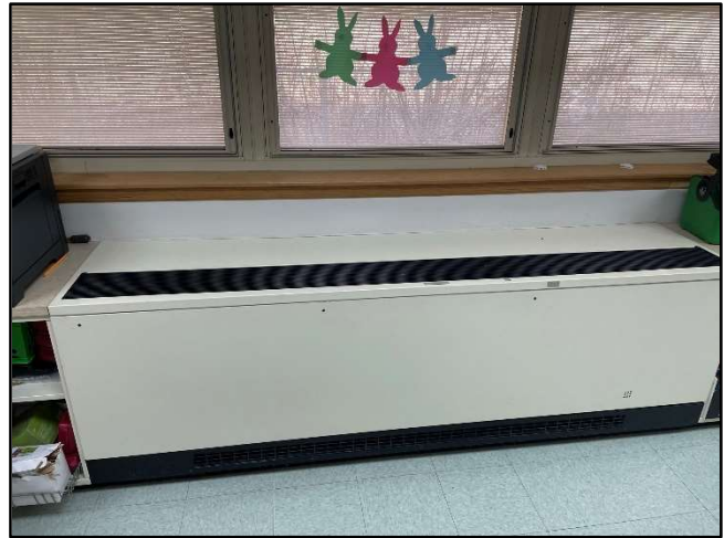
Existing unit ventilators at Slocum Skews and Shaler Academy
