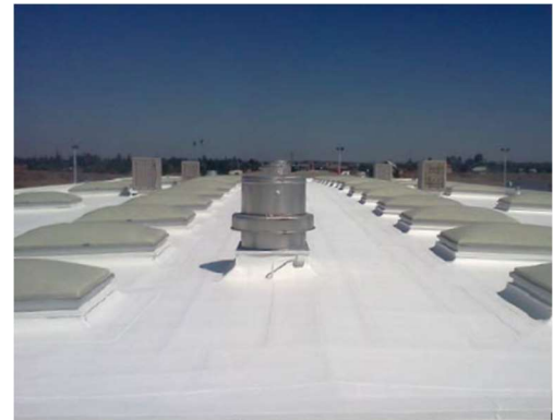
Single Ply Membrane Roof Restoration
