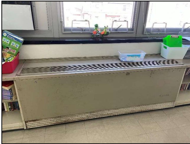
Existing unit ventilators at Slocum Skews and Shaler Academy
