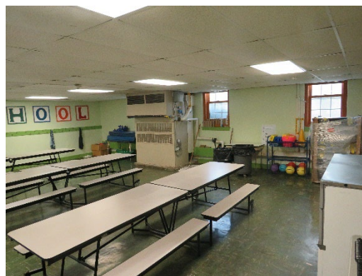
Existing Lighting at Samuel Smith ES
