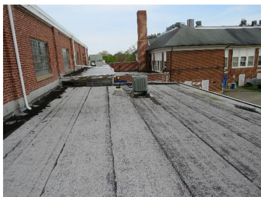
Samuel Smith ES – Roof Replacement
