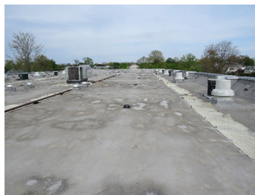
Samuel Smith ES – Roof Replacement
