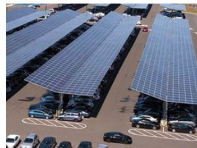
Typical Parking Lot Solar Array
