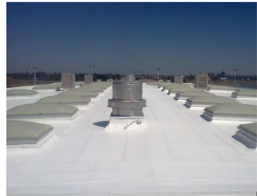
Single Ply Membrane Roof Restoration
