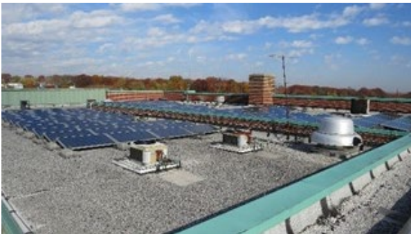
Lincoln ES - Building Envelope
