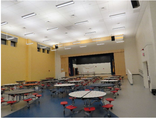
Lighting at Kennedy Elementary School
