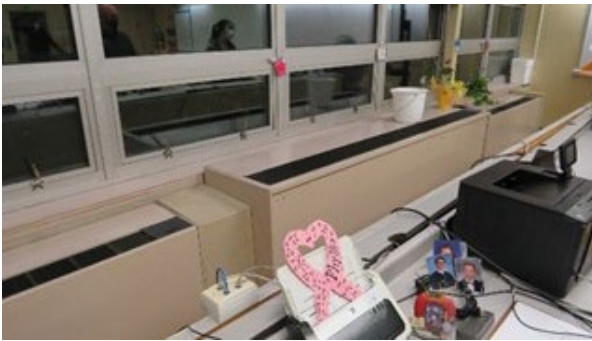
Washington MS – Typical Unit Ventilator
