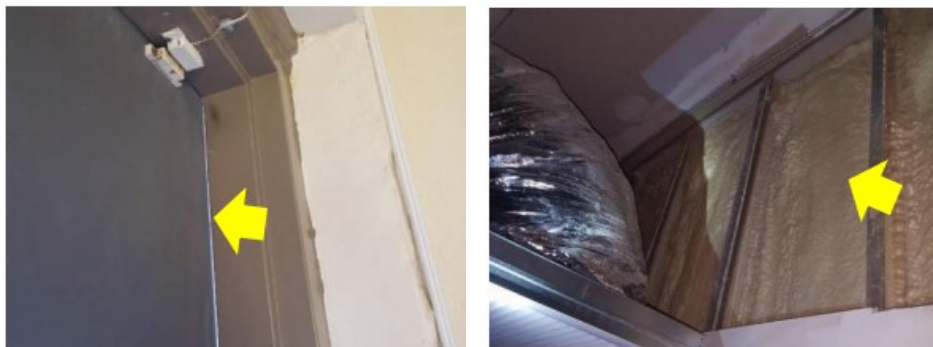
Existing Conditions at the Administration Building
