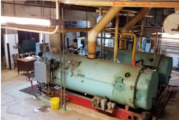
Existing steam and hot water boilers at Schuyler Elementary School
