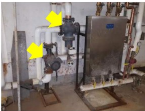
Uninsulated pipe and valve insulation at Lincoln Middle School
