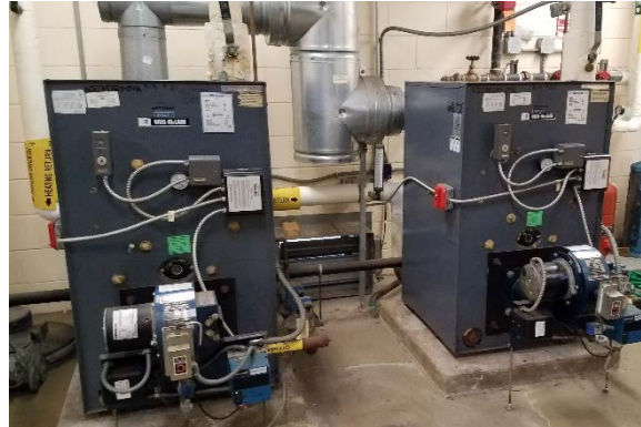
Existing steam and hot water boilers at Schuyler Elementary School
