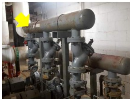
Uninsulated pipe and valve insulation at Lincoln Middle School
