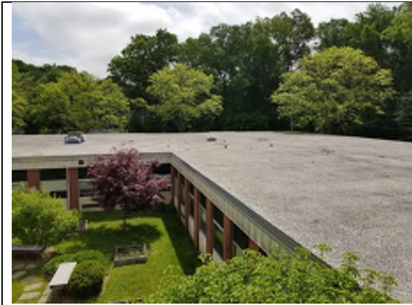
Flat Deck Roof
