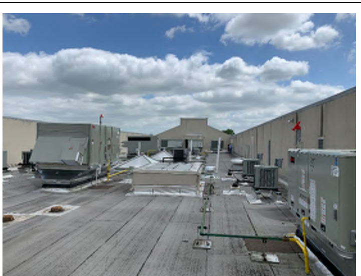
Flat Section of Roof
