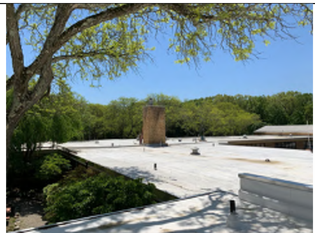
Flat Deck Roof
