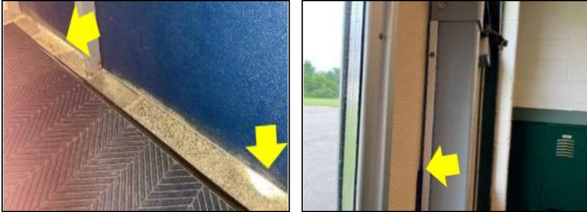
Existing Conditions at Ramapo HS and Indian Hills HS
