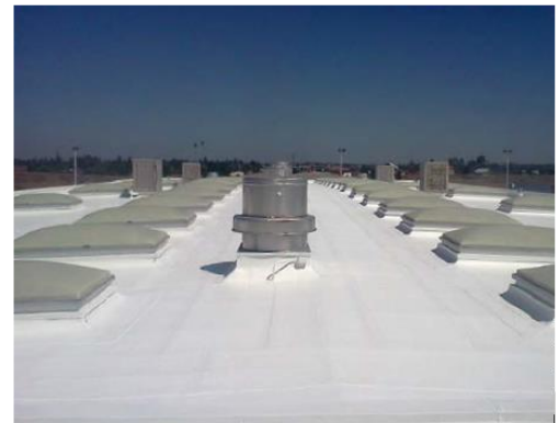
Single Ply Membrane Roof Restoration
