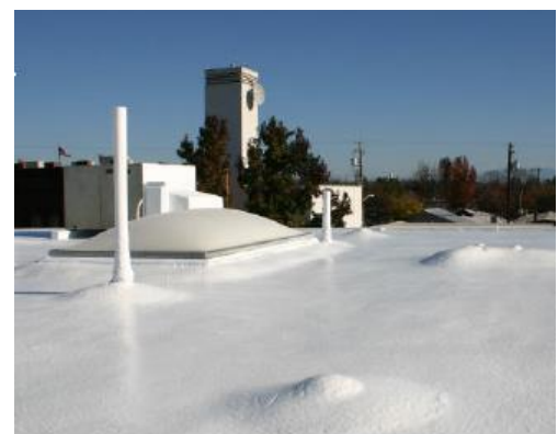
Spray polyurethane foam Roof Restoration
