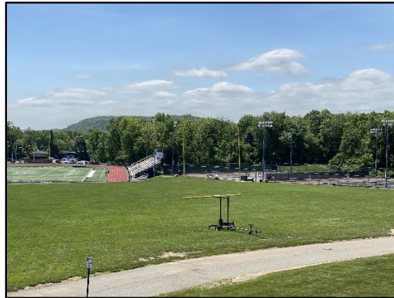
Existing Field Lighting at Ramapo HS
