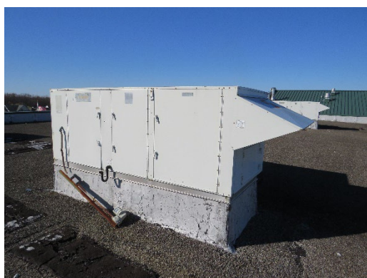
Governor Charles C. Stratton School - RTU
