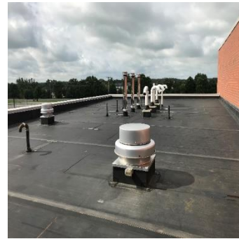
Image 4 Black membrane on roof
