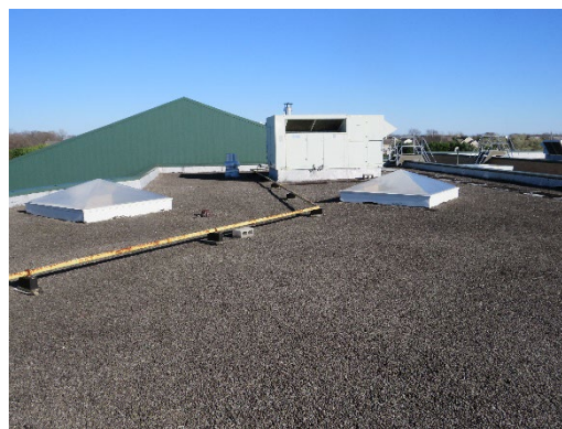
Governor Charles C. Stratton School – Roof Replacement
