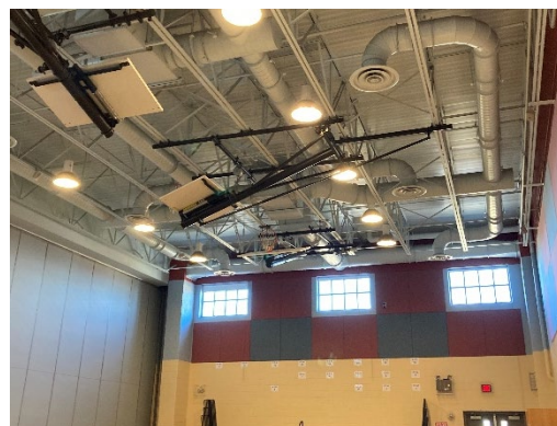
Walter Hill School – Multi-purpose Room
