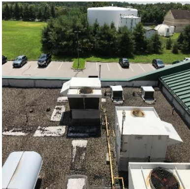
Image 10 Units on flat roof
