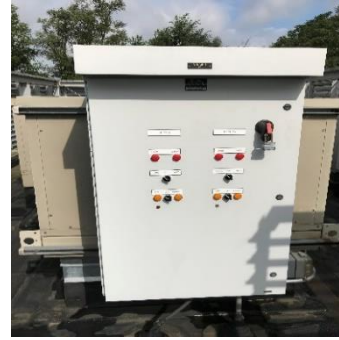
Image 10 AHU controls
