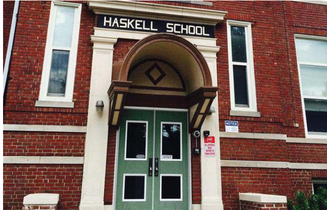
Figure 3: Haskell Elementary School
