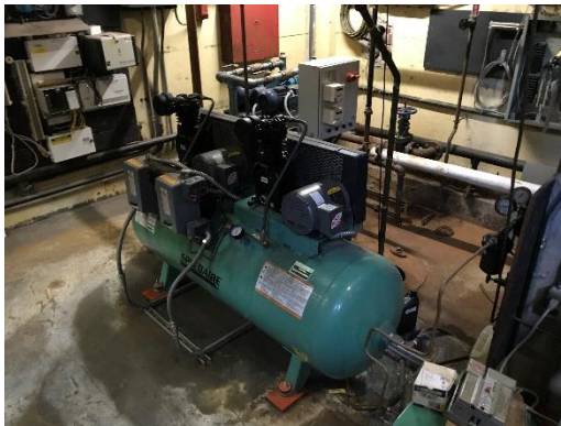
Middle School Pneumatic Controls Compressor
