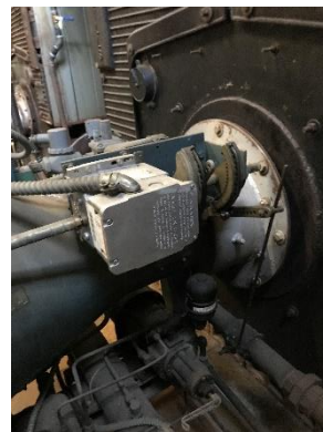
Linkage-Type Burner Controls
