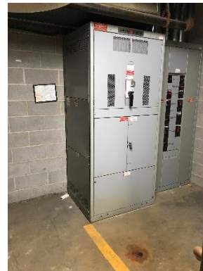
Middle School Electrical Switchgear
