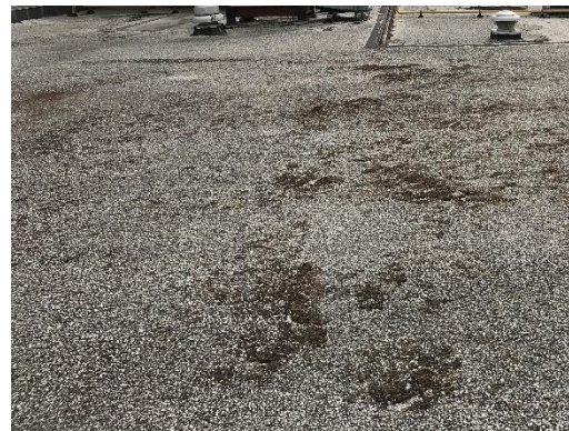
High School Roof Debris Buildup
