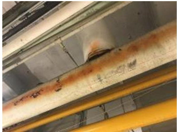
Examples of Uninsulated Piping
