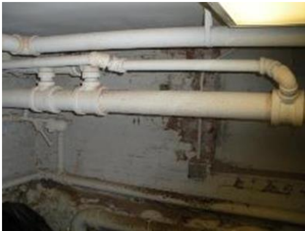
Examples of Uninsulated Piping
