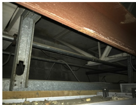
Overhang Air Sealing – there is no barrier separating the exterior overhang (area beyond metal framing) from the conditioned interior space (Rosa L. Parks HS).
