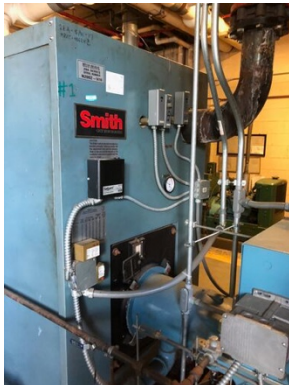
Gas Fired Boiler
