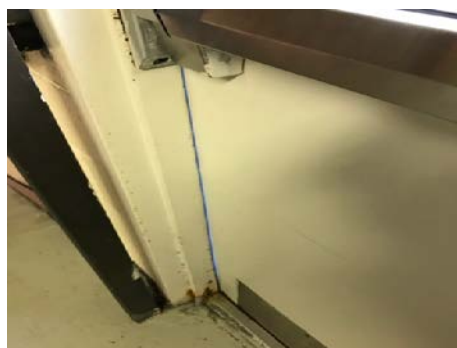
Door Weather Stripping – daylight showing through the sides of the door is a clear indicator that there is not a tight weather stripping seal (Silk City 2000 Academy).
