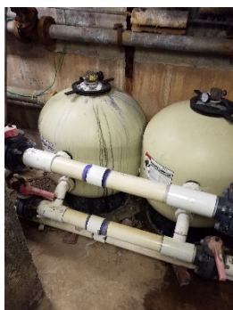
Existing Pool Filters - Norman S. Weir
