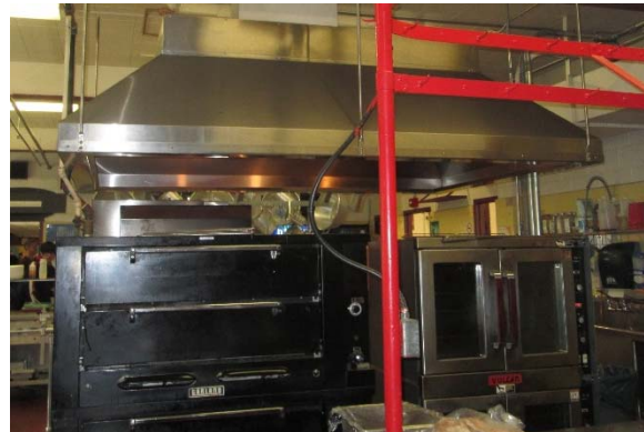
Existing Kitchen Hood
