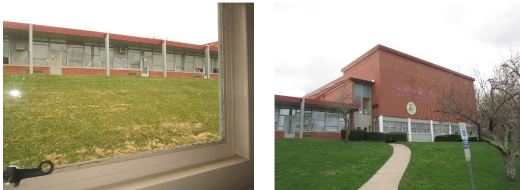
Window Replacement Opportunities
