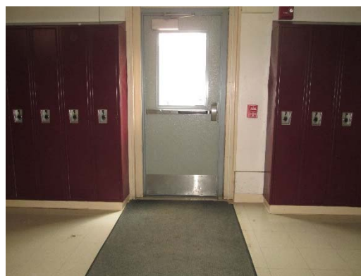
Door Replacement Opportunities
