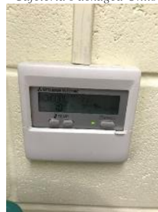
Programmable Thermostat for Split Units
