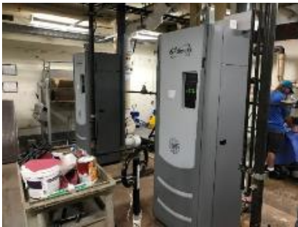
Condensing Boiler
