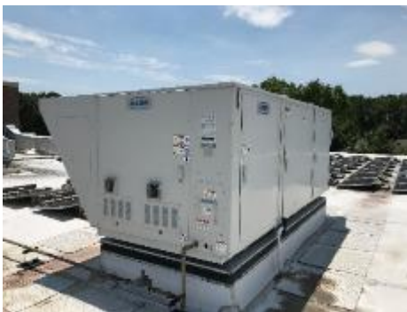
Packaged Unit with Gas-fired Furnace
