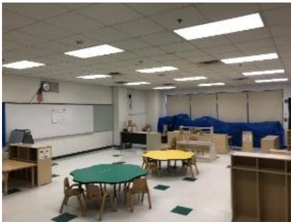
Lighting in the Classroom
