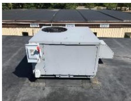
Packaged AC and Heater
