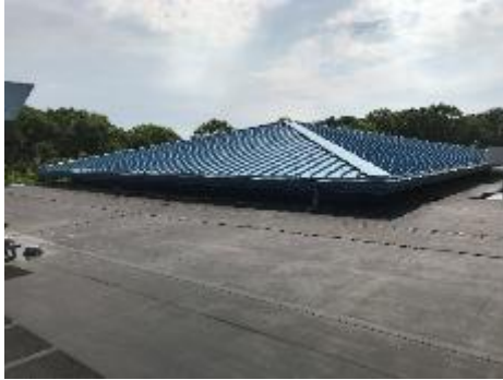
Pitched Metal Roof
