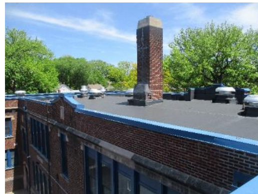
Roof – E. Roy Bixby Elementary School
