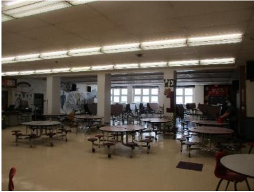
Existing Lighting at Bogota Jr. and Sr. High School
