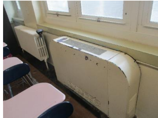
Unit Vent Replacement– Bogota Jr.and Sr. High School
