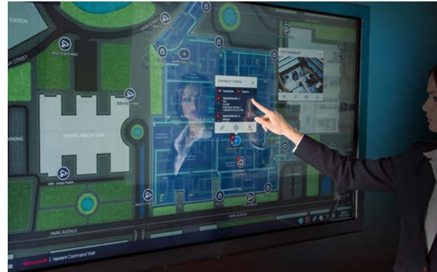
HVAC Equipment Control
