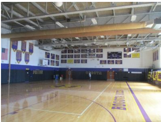
Lighting Control Space at Bogota Jr. and Sr. High School
