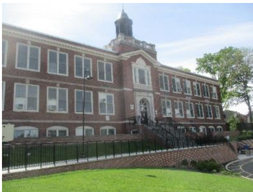
Window AC Units – Bogota Jr. and Sr. High School
