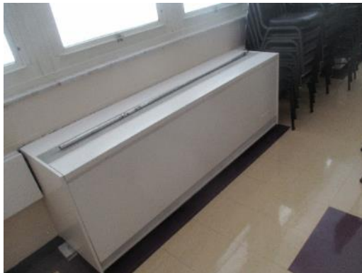
Unit Vent Refurbishment– Bogota Jr.and Sr. High School
