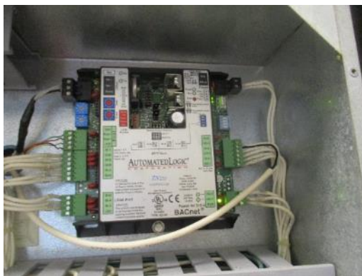
Existing Controls – E. Roy Bixby Elementary School
