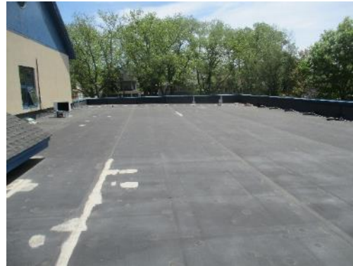
Potential Roof Solar – Lillian M. Steen Elementary School
