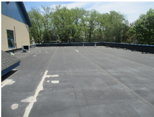
Roof – Lillian M. Steen Elementary School
