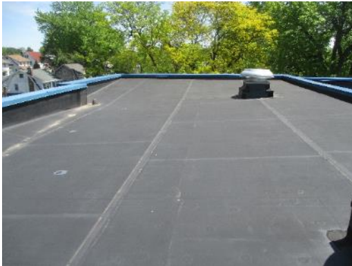
Potential Roof Solar – E. Roy Bixby Elementary School
