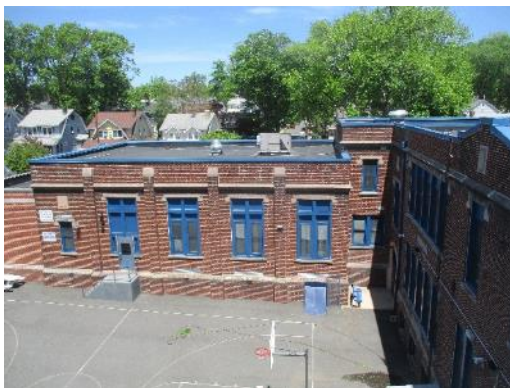
Building Envelope – E. Roy Bixby Elementary School
