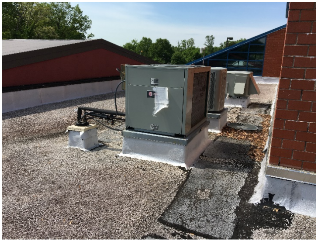
Existing split system AC units at Switlik Elementary School
