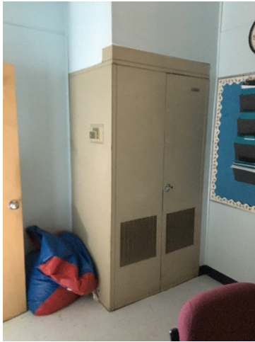
Existing electric/DX unit ventilators at Switlik Elementary School
