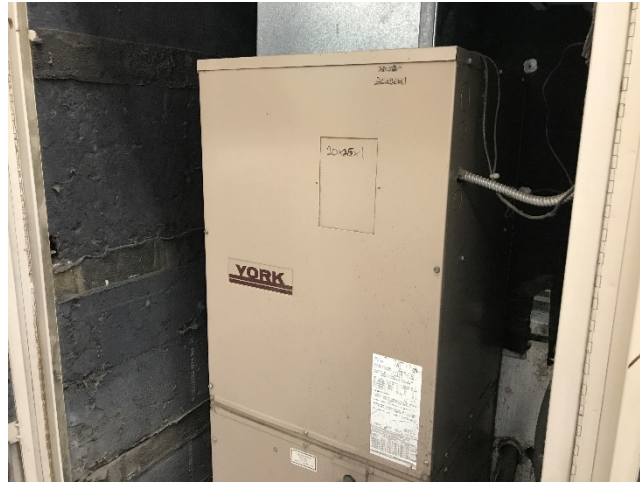
Existing electric/DX unit ventilators at Switlik Elementary School
