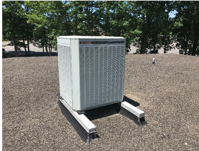
Existing split system heating and cooling unit at the Administration Building
