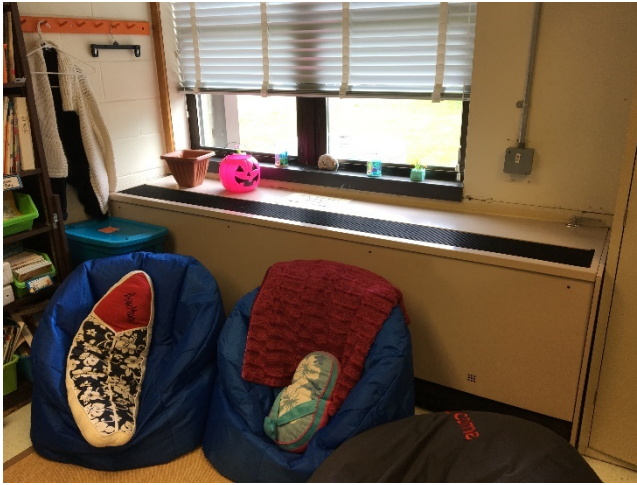
Existing HW/DX unit ventilators at Rosenauer Elementary School
