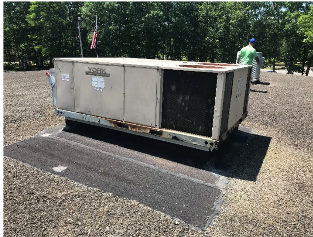
Existing roof top unit at the Administration Building
