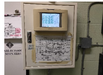
VRF Controller Head Unit
