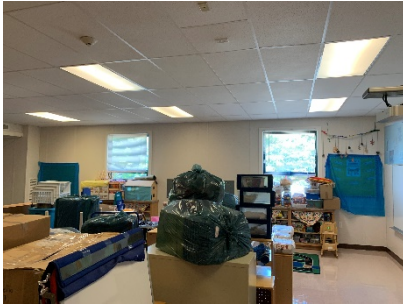
Early Childhood Center Classroom Lighting
