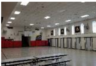
Westbrook MPR Lighting
