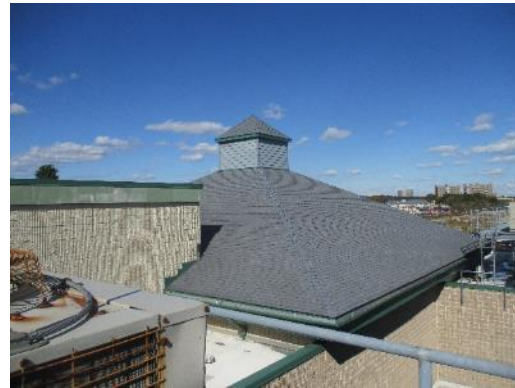
Building Envelope – Roberts Academy 30
