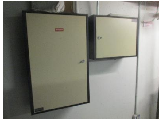
Existing Controls – Edreira School 26
