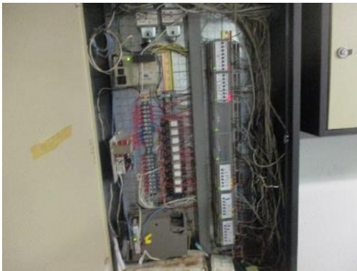
Existing Controls – Edreira School 26
