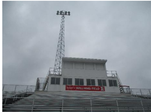
Williams Field Stadium Lights
