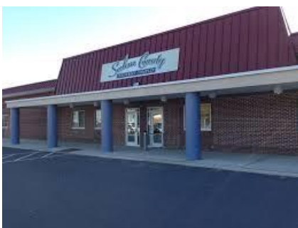
Figure 9: Main County Office Building
