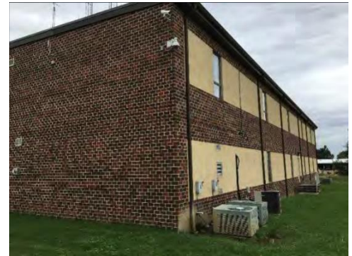
Emergency Services Building
