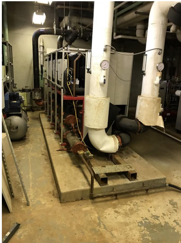
Figure 3: Multistack Chiller
