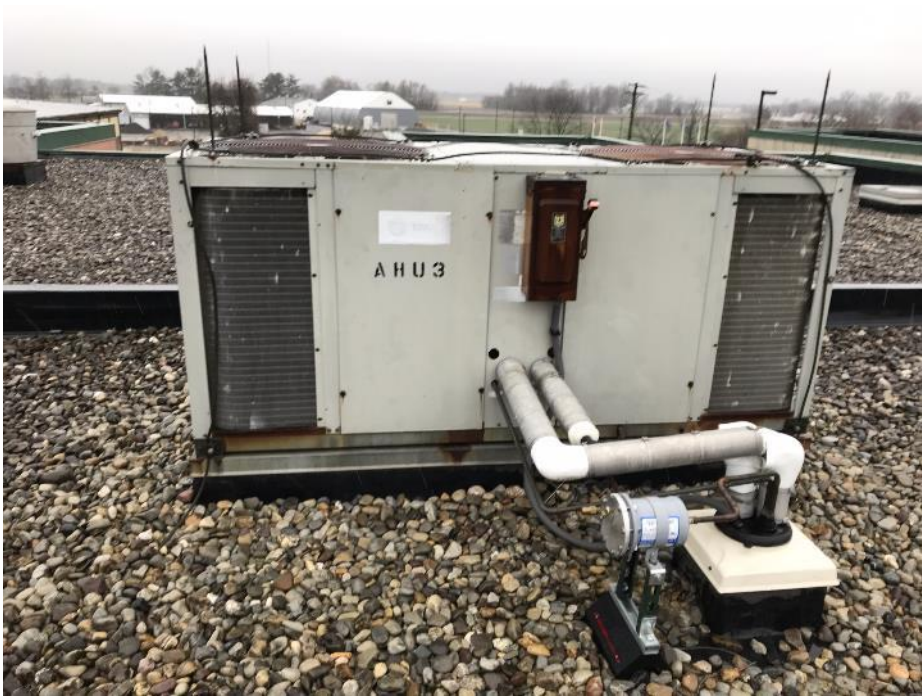
Figure 3: AHU-5 Heatcraft Air-cooled Condenser (top), AHU-3 Trane Air-cooled Condenser (bottom)
