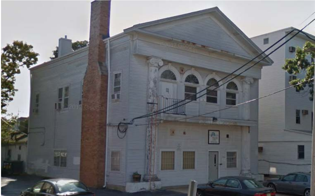
Figure 24 IT Center Building Exterior
