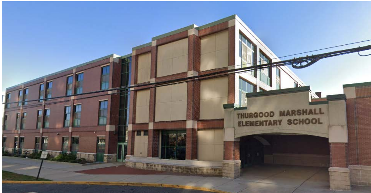
Figure 19 Thurgood Marshall Elementary School Building Exterior
