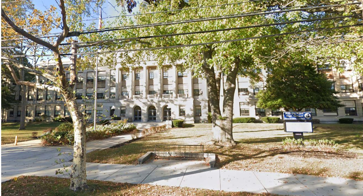
Figure 2 Asbury Park High School Building Exterior
