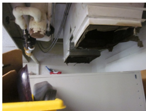
Removed Cafeteria AHU – Mohawk ES
