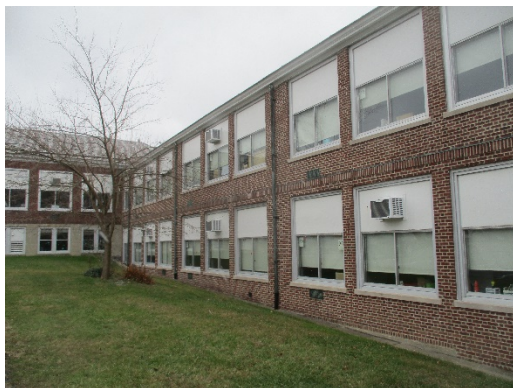
Building Envelope – Mohawk ES
