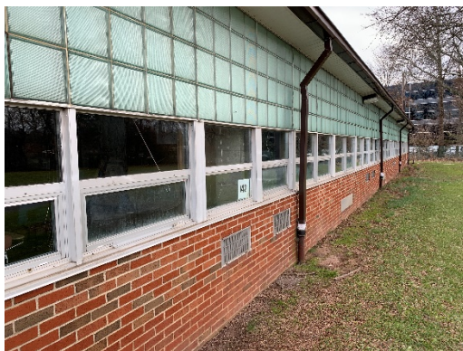
Windows at Piscataway HS
