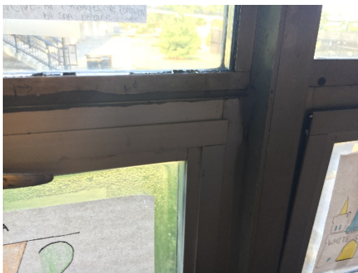
Windows at Piscataway HS
