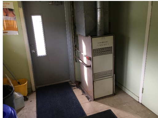
Ethel Road Complex Furnace
