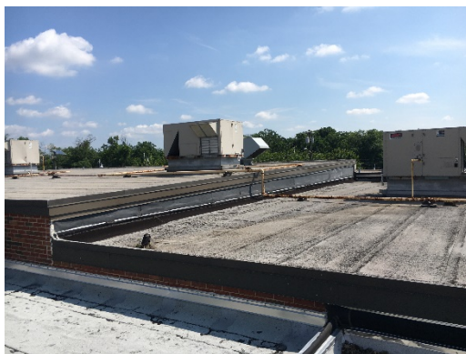
Roofing at Piscataway HS
