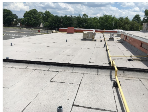
Roofing at Eisenhower ES
