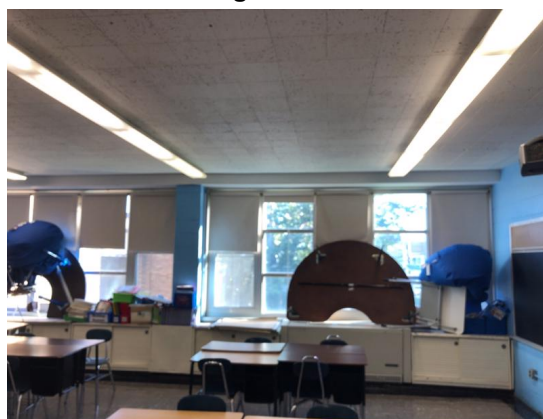
Corridor and Classroom Lighting
