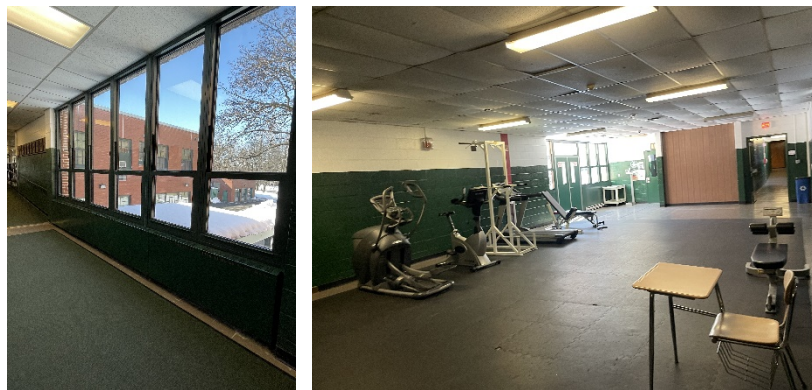
Existing air sealing opportunities at Passaic Valley Regional HS
