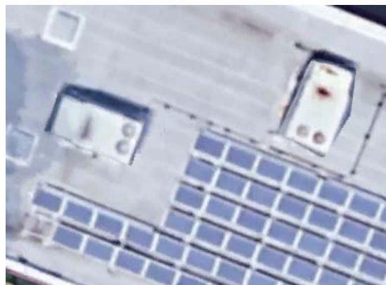
Existing RTUs at Passaic Valley Regional High School
