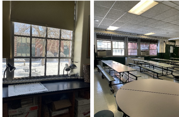
Existing windows at Passaic Valley Regional High School
