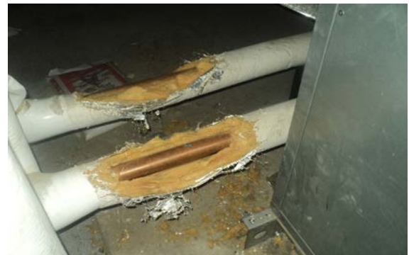
UNINSULATED HOT WATER PIPING
