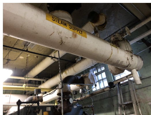
Damaged pipe and valve insulation at WOK Middle School and George Washington Elementary School
