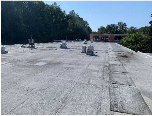
Watchung Hills RHS – Potential Roof Solar
