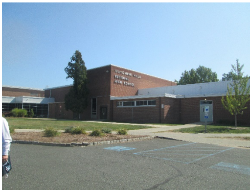
Windows – Watchung Hills RHS
