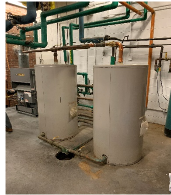
DHW - Kitchen Storage
