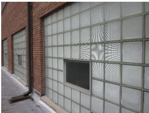
Building Envelope – Watchung Hills RHS
