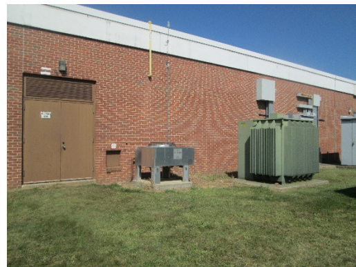
Building Envelope – Watchung Hills RHS
