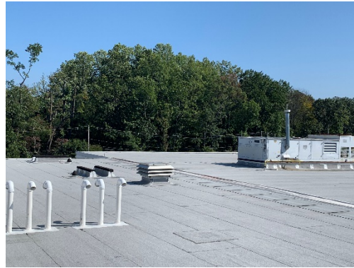
Watchung Hills RHS – Potential Roof Solar
