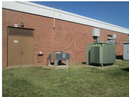
Existing Lighting Outdoor Fixtures
