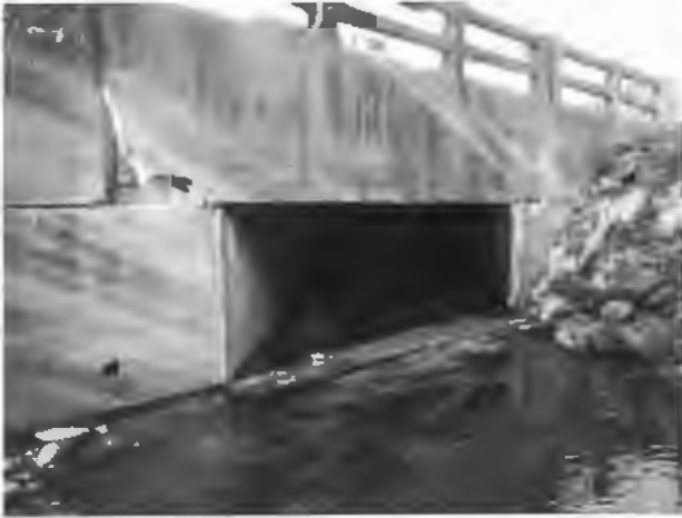
Photo ID: 1 Direction: W
