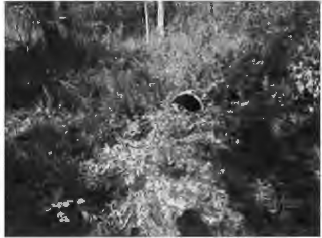
Photo ID: WET-A Direction: N
