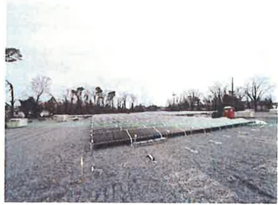
Figure 10. More racking and modules installed April 6, 2022
