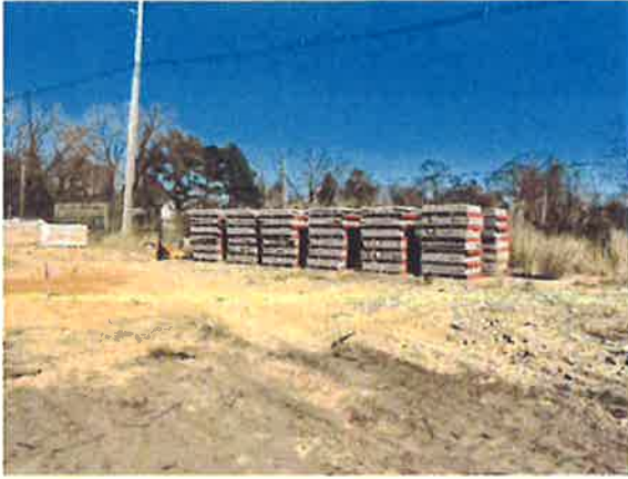
Figure 5. Ballast blocks for racking system delivered March 21, 2022
