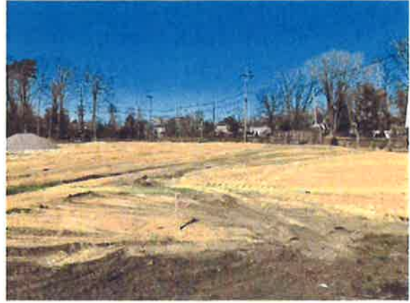
Figure 6. Preparing site for solar mobilization March 21, 2022
