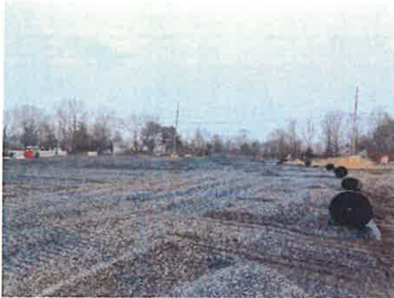
Figure 11. More gravel being placed for module installation April 7, 2022
