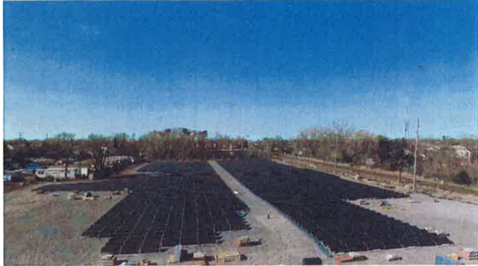
Figure 13. Solar racking and modules installed at 80 % April 26, 2022
