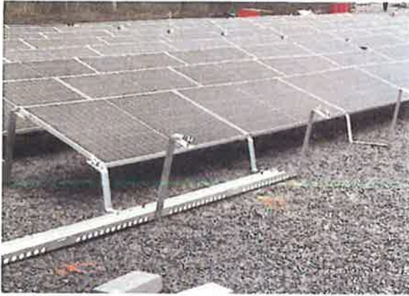
Figure 9. Racking and modules beginning to be installed March 24, 2022
