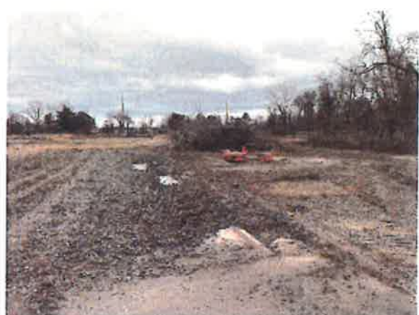
Figure 4. Site clearing January 17, 2022
