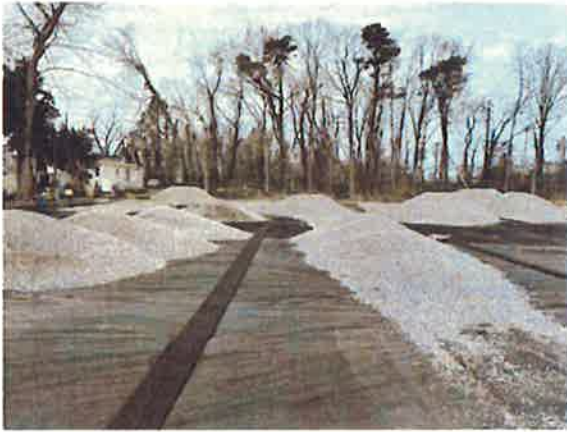
Figure 7. Prepping to lay down gravel March 23, 2022
