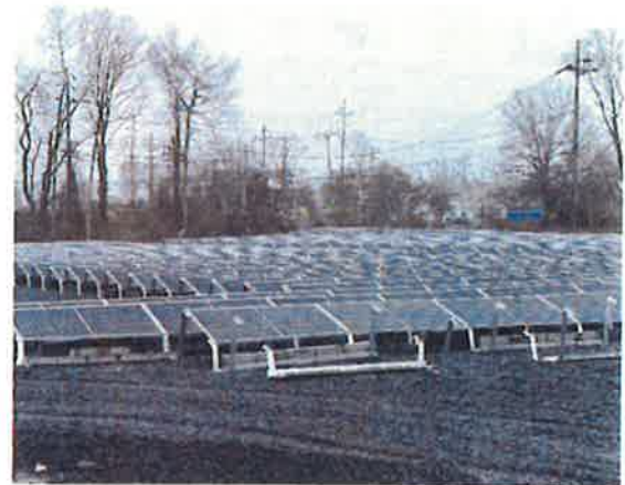
Figure 12. Solar racking and modules being installed April 7, 2022
