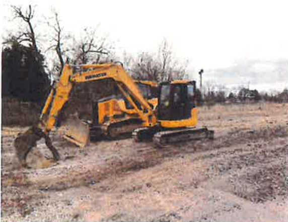
Figure 3. Site clearing January 17, 2022
