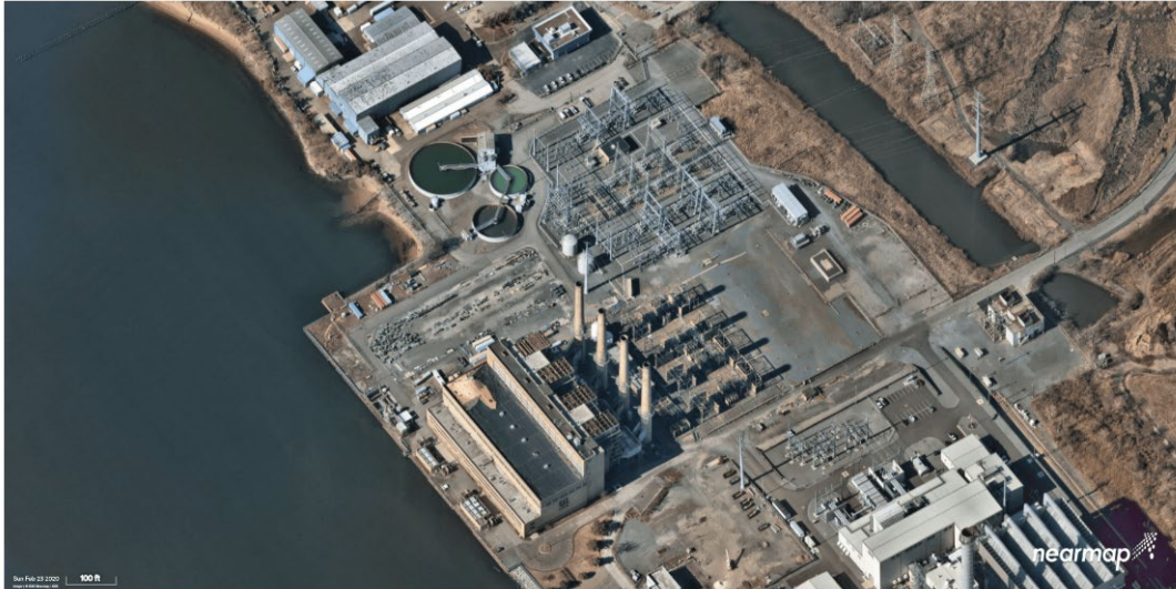
Figure 2 Existing Sewaren Site
