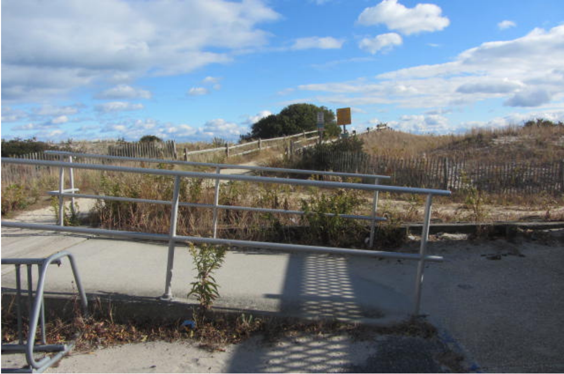
3. View of Easement Lot (Lots 137) from 35 th Street Terminus facing Southeasterly
