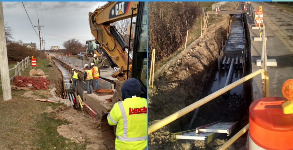
Underground duct work installed via trenching
