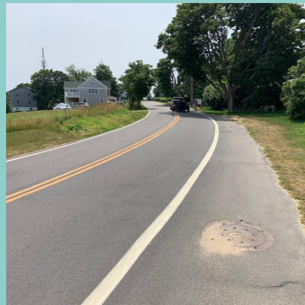
Post-construction pavement restoration
